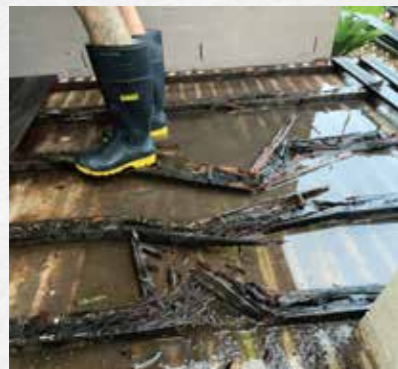
2 year old H3 treated pine deck frame on concrete
